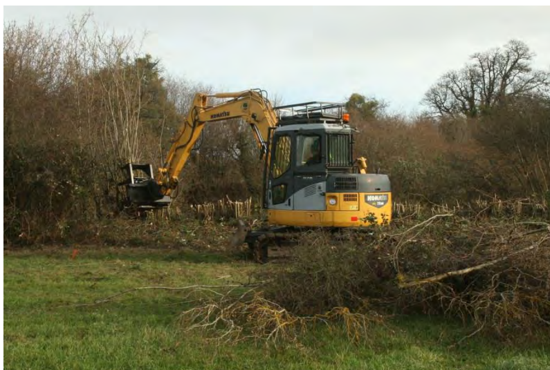
Figure 3.6. Excavator mounted 10"/250mm Dymax tree shears coppicing Hedge 21 at Elm Farm
